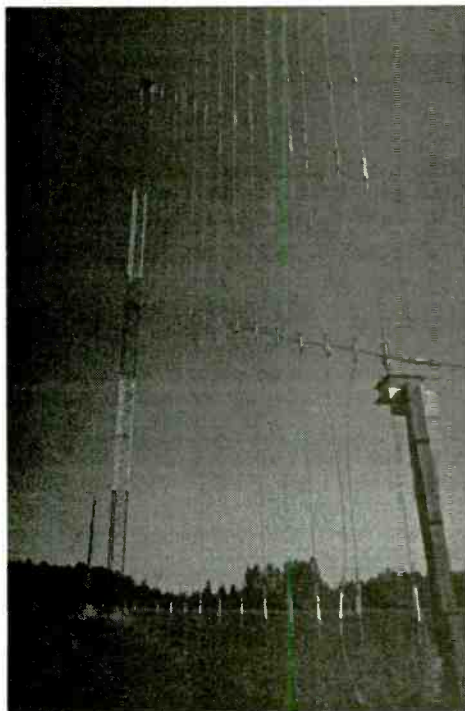
View of one of the curtains on the vertical log periodic antenna.
