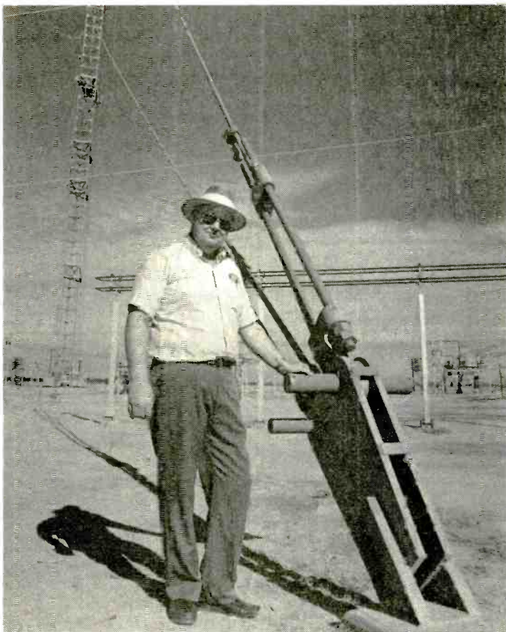
Station manager Lynn Smith stands next to one of the many anchors that support the curtain array antenna.
