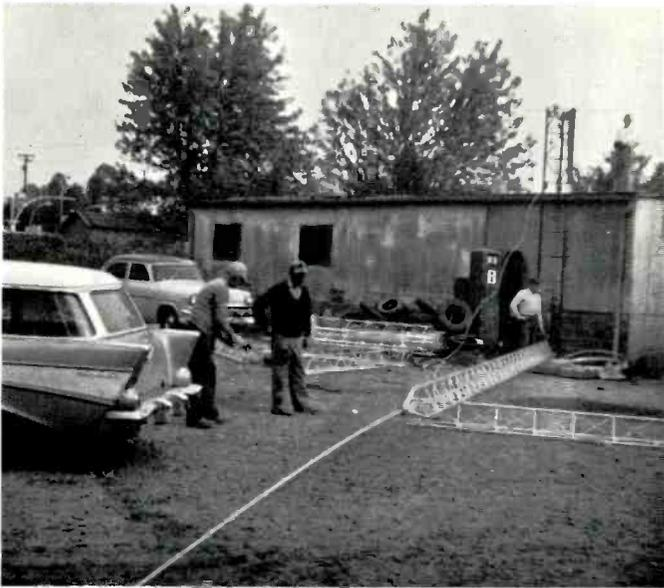
30 foot top section of tower and antenna erected and ready to be lifted into Kwik-Up Erector.
