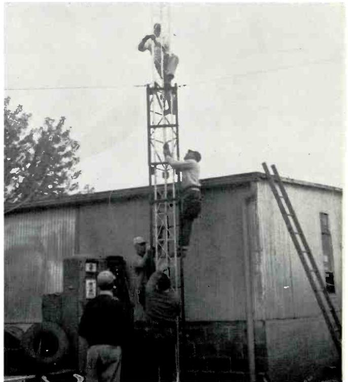
Guys are attached to section of tower already lifted above ground before the next section is cranked into place. This is as far as a man ever gets off the ground.
