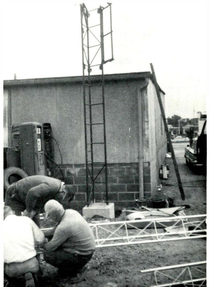
Kwik-Up Erector Kit installed on tower base and guyed, ready for first 30 feet of tower to be slid inside frame.
