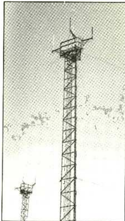
Here's what an FAA Traffic Control Center directional antenna at a remote location looks like.
