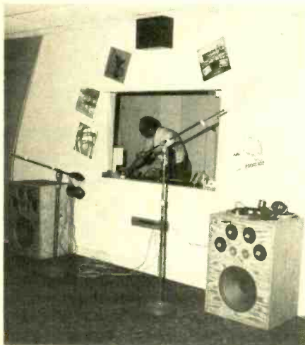
Asbury Records' studio features heavily carpeted flooring and semi curved walls (left) to inhibit sound reverberation. The glass pane in the studio-to-control room window is tilted slightly for additional protection from reverb. Microphones are attached to booms to insure exact positioning during recording sessions. The dual multi-coned speakers on either side of the control room window are used for playback of recordings. A row of microphone connectors seen between the two boom mics lead directly to the control room mixing console on the other side of the wall. Album covers serve as decoration around the control room window.
