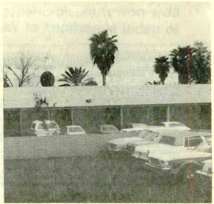
Microwave dish on building top connects studio to transmitter approximately four miles away.
