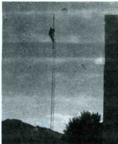
Gin pole being raised up to last stage to raise final 10 foot pole to top to be inserted in tower top.
