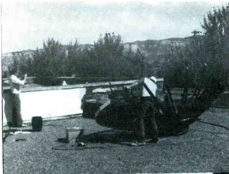
12 foot mesh dish takes two people better part of a day to assemble. Local Cortez satellite expert lift sites in true South and was instrumental in helping getting the operation on the air, as well as getting the satellite dish oriented and working.
