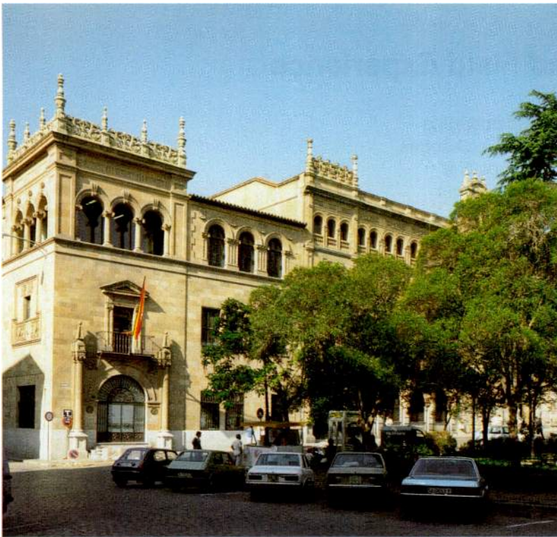
Exchange building in Salamanca which houses Spain's first System 12 digital exchange. The capacity of the exchange is 10000 subscriber lines.
