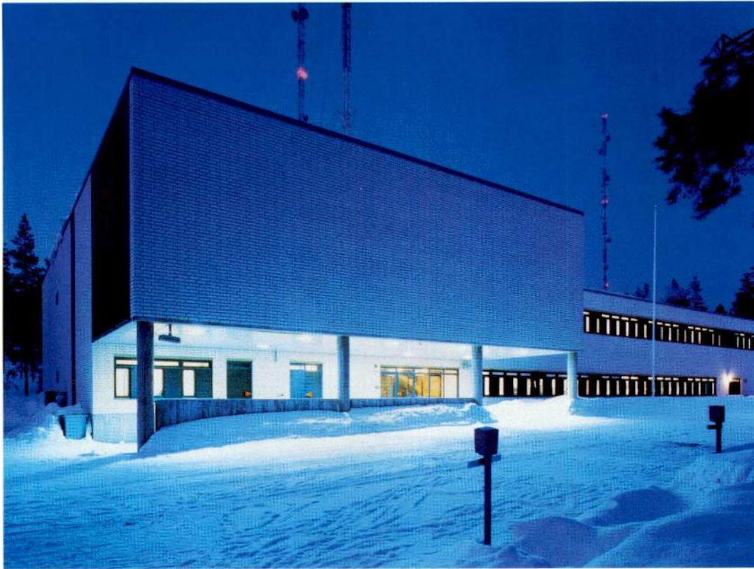
Building housing the Seinajoki System 12 digital exchange in Finland.
