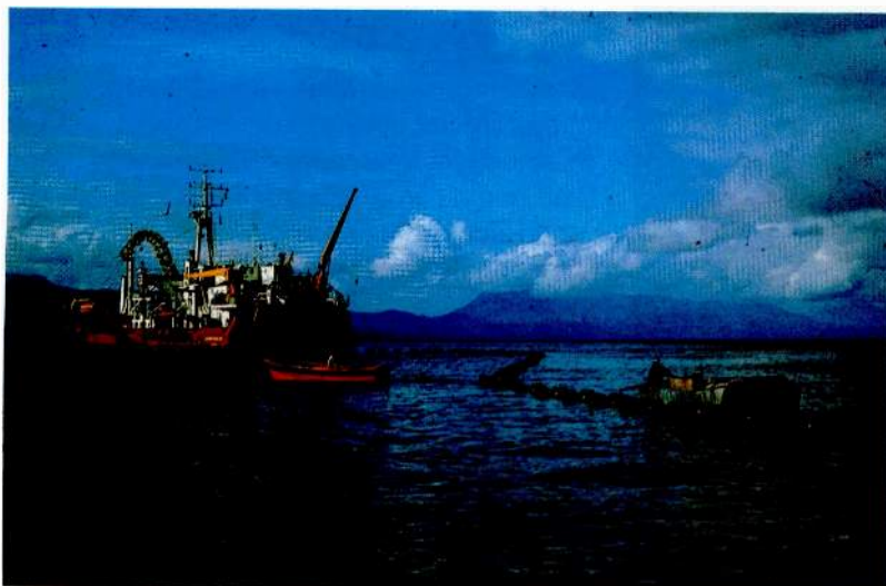
Floating a cable end ashore.
