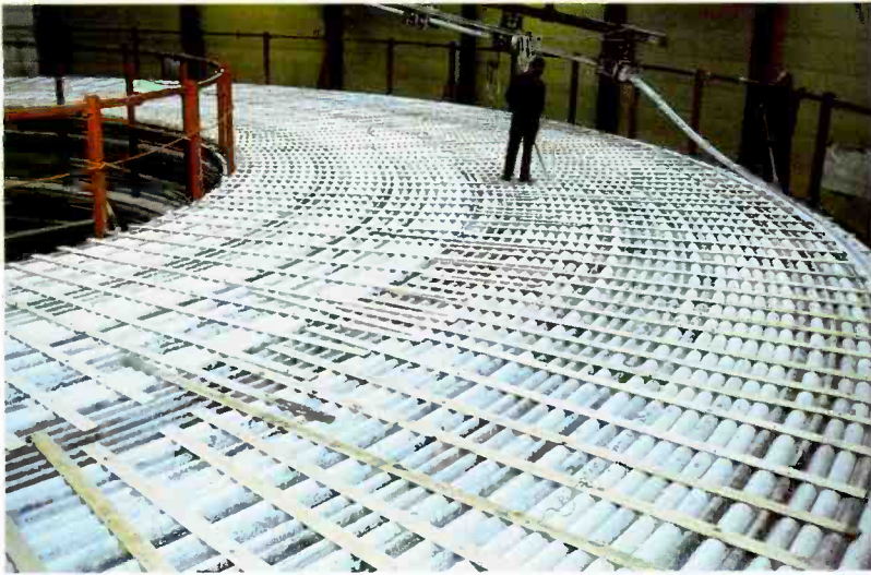
Turntable at STK's submarine cable plant; it can hold up to 6500 tonnes of cable.
