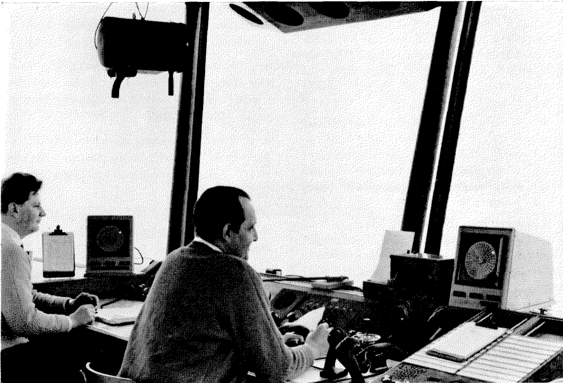
Figure 16—Installation of two slave light indicators in the control tower at an airport.
