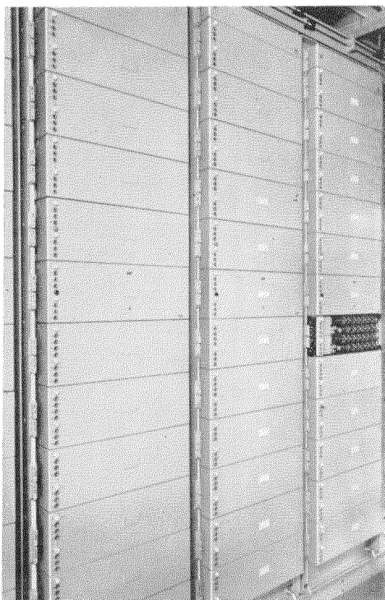
Figure 8---Adapter circuit for 2-wire/4-wire or 4-wire/4-wire connections, with hybrid coils.
