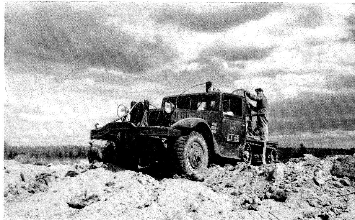
Figure 6—Half-track vehicle used for laying cable in trench.
