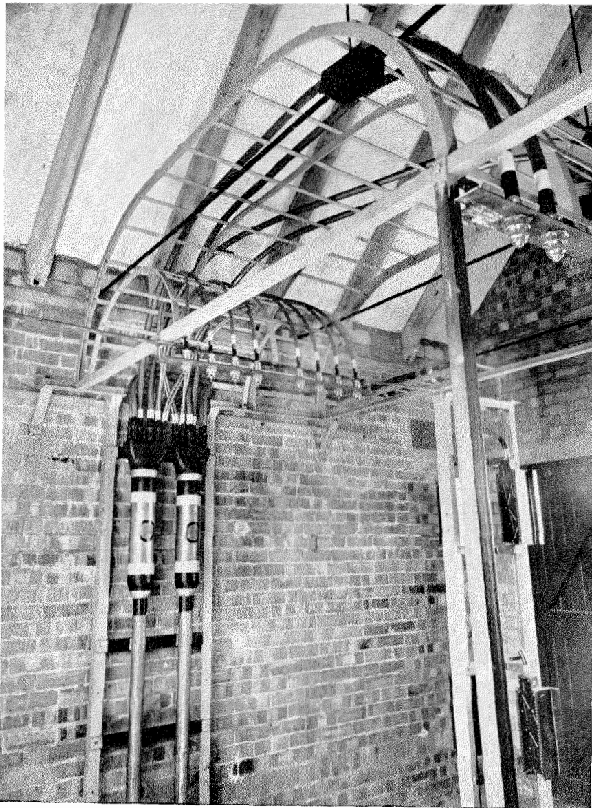
Figure 7—Cable terminations.
