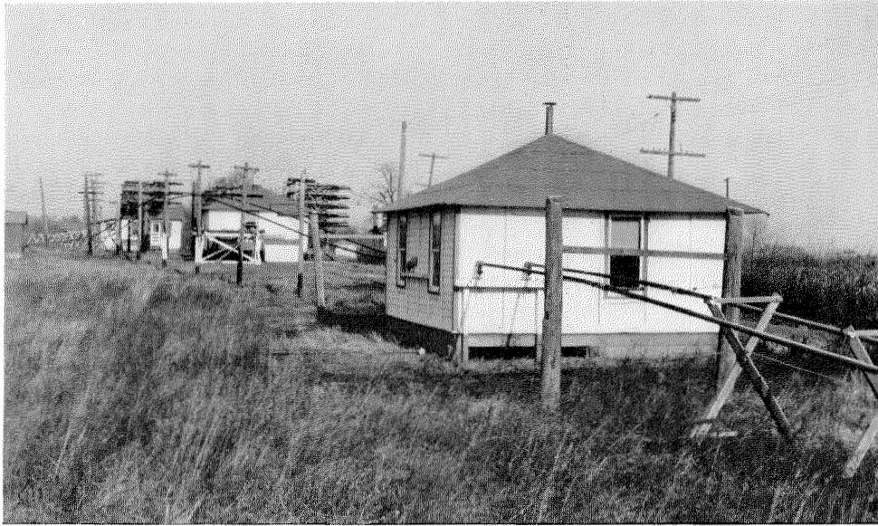
Figure 4—Phoenixville Installation Showing Conductors Entering Test House.
