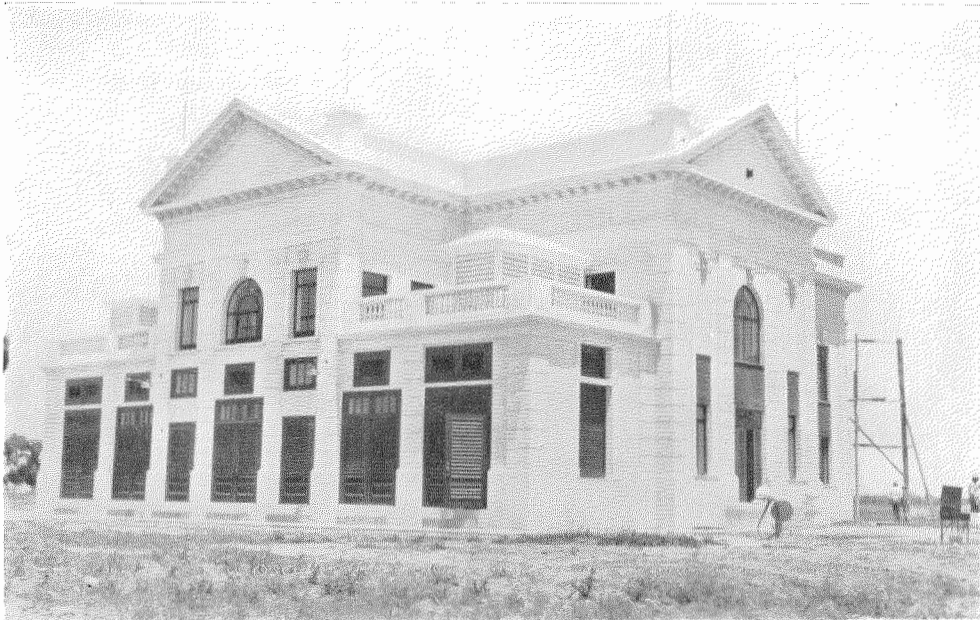
Transmitter Building at Hurlingham, Rear View
