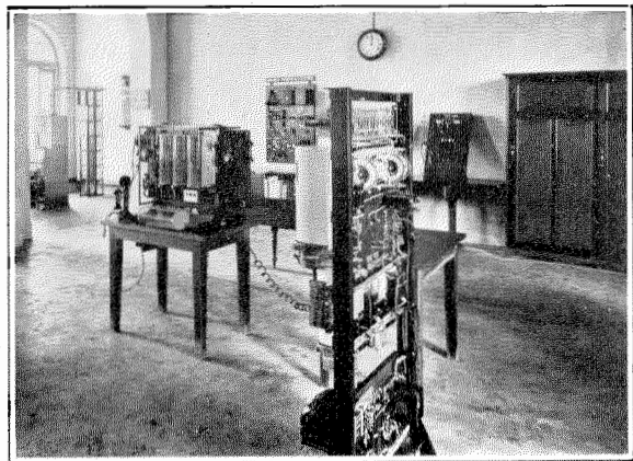
Figure 5—Telegraph Department Training School. Telephone and Telegraph Section. Automatic demonstration sets in foreground. Model office in rear at left.
