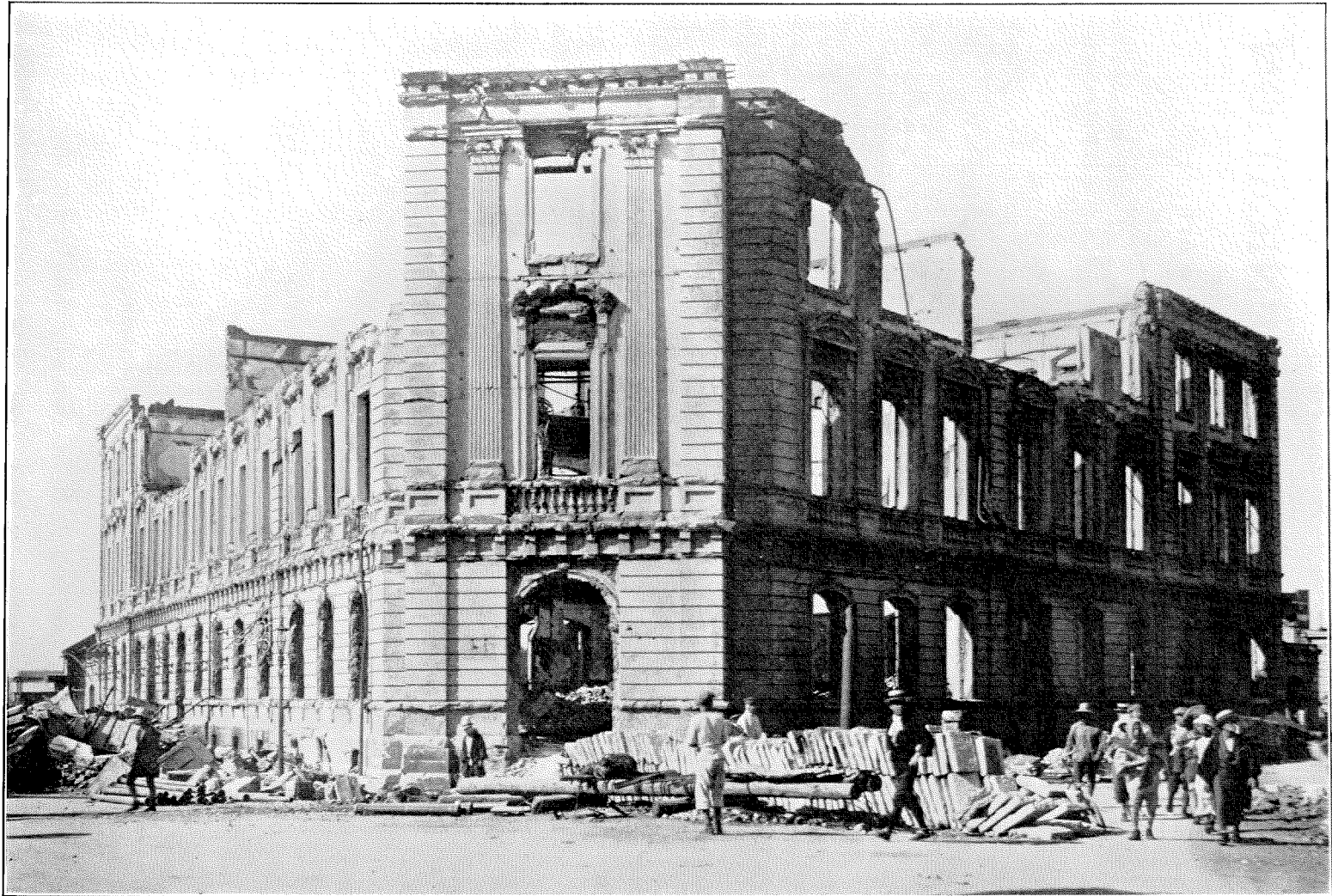
General View of Tokio Central Telegraph Office After Fire
