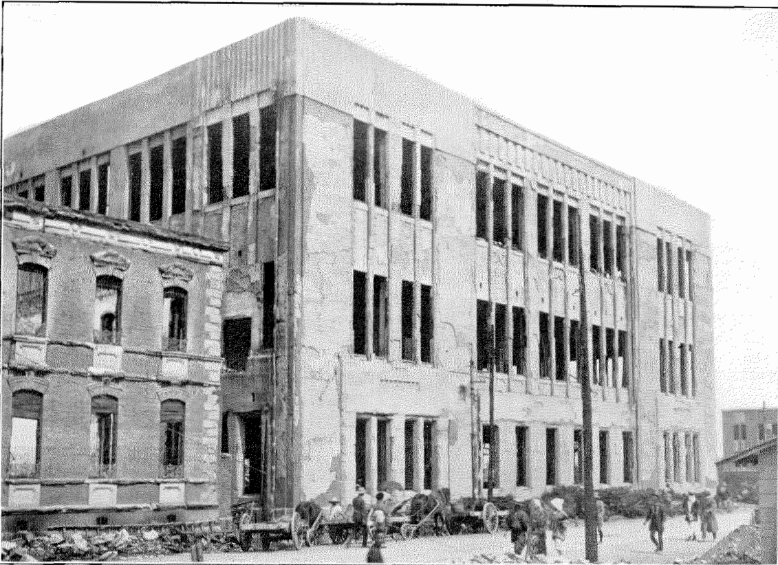
Figure 8—Outside View of Building After Fire, in which were located two units of Telephone Central, Hamacho and Horidome, Tokio. Reinforced concrete building to be used again as Common Battery Office. Brick building to left is Central Naniwa
