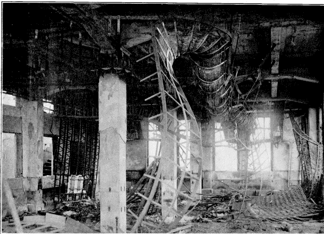
Figure 10—Ruins of Cable Room After Fire in Telephone Central Horidome, Tokio
