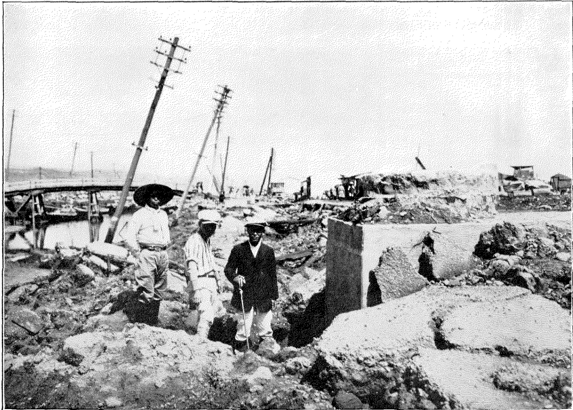
Figure 17—Manhole Near River Bank in Yokohama Remained Unsunken. Head of Manhole Projecting Above Road Surface
