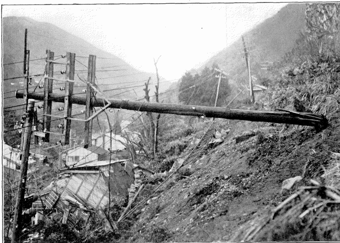
Figure 18—Disaster of Pole Line Near Hakone. Longer Poles are for Power and Lighting. Smaller Ones for Telephone
