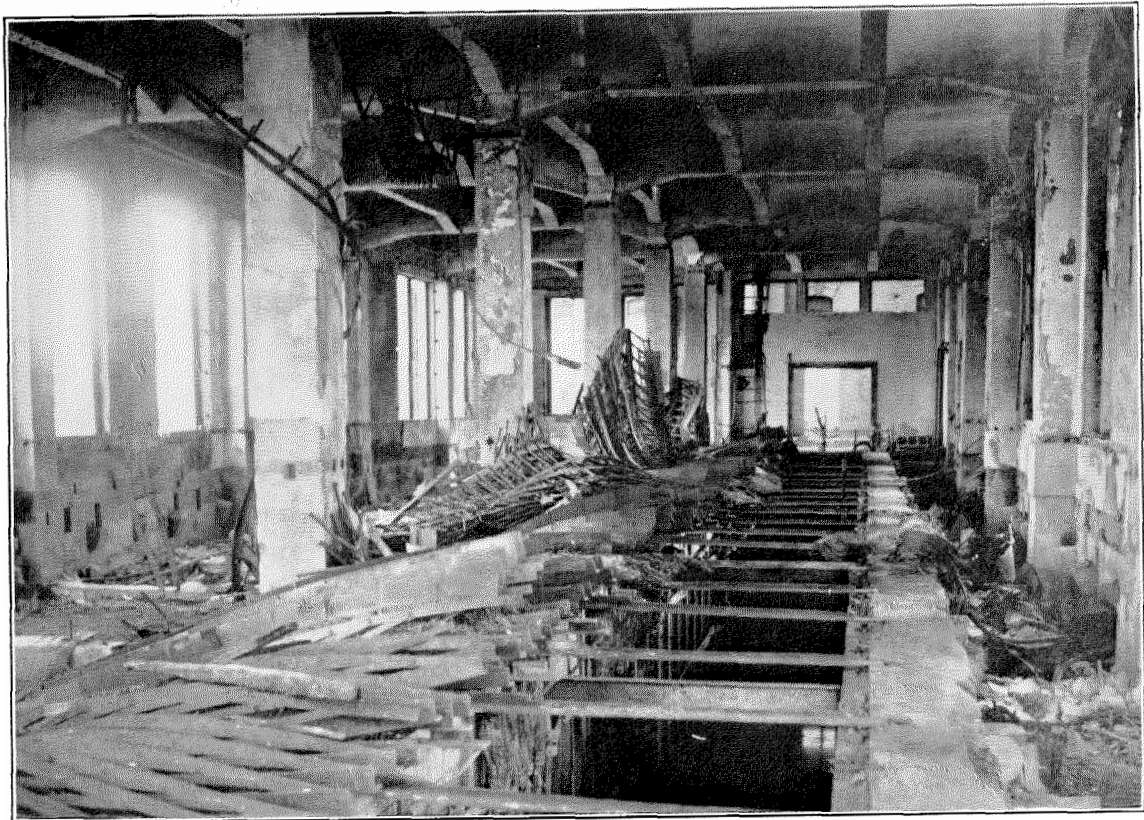
Figure 12—Ruins of M. D. F. and Office Manhole After Fire in Telephone Centrals Hamacho and Horidome, Tokio
