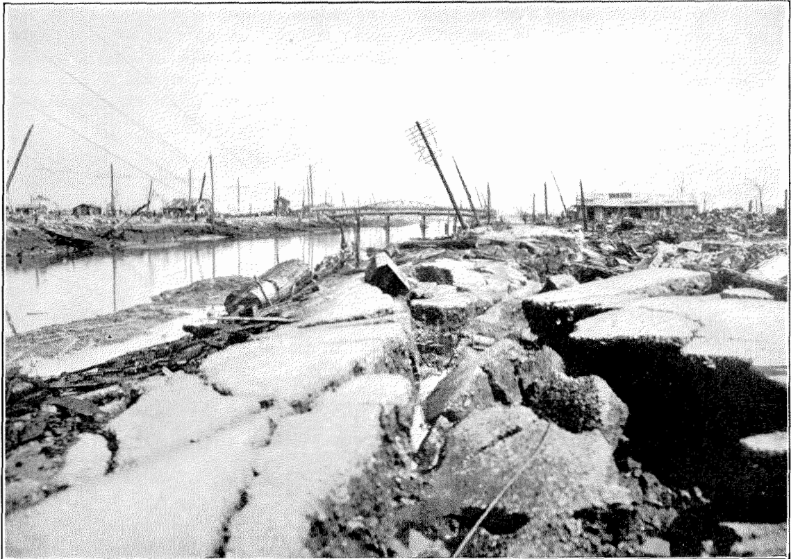
Figure 1—Cracks in Ground Near a River in Yokohama—Telephone Pole Near Center of Picture
