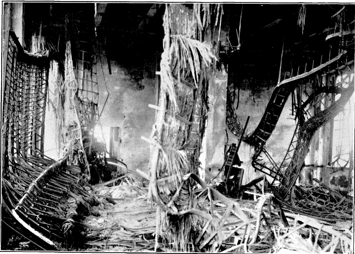
Figure 9—Ruins of Cable Room After Fire in Telephone Central Hamacho, Tokio
