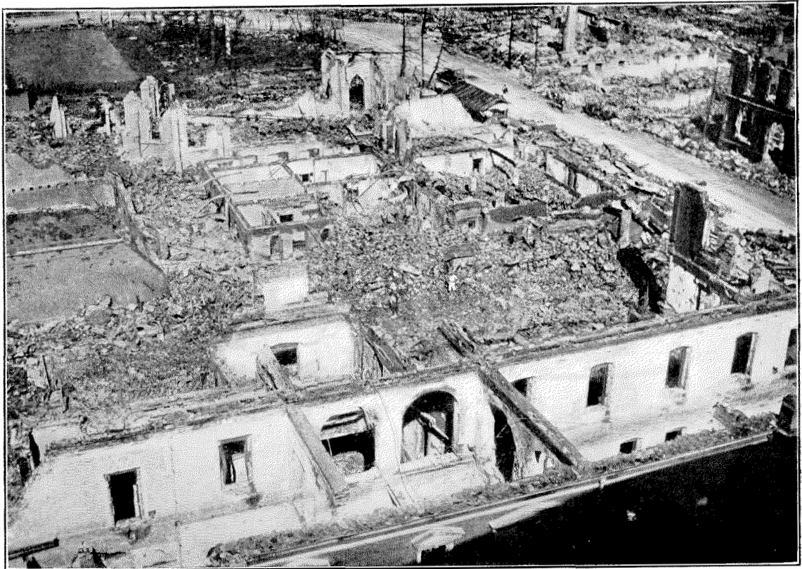
Figure 5—General View of Ruins of Telephone Central Honkyoku, Yokohama
