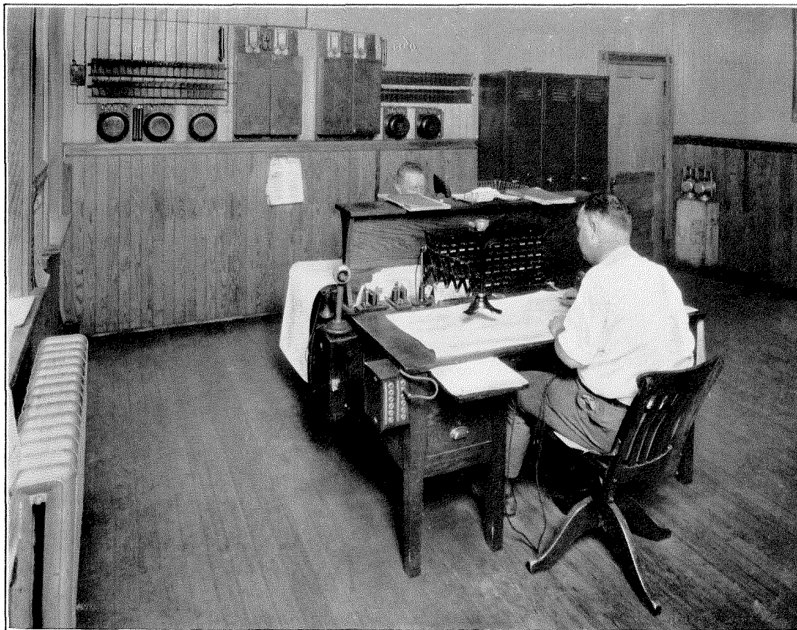
Figure 18—Train Dispatcher's Office. Loud Speaking Equipment Installation
