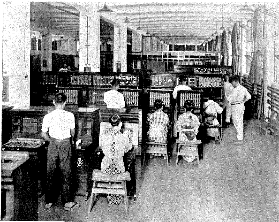
Nippon Electric Company—Switchboard Assembly
