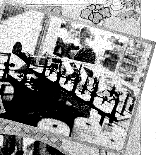
Winding paper and tinfoil to make telephone condensers
