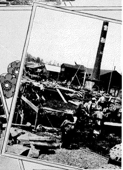
Inside the compound preparing for new building construction
