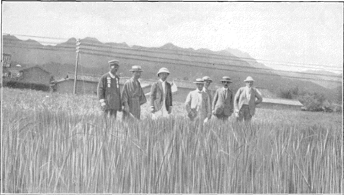
Survey Party on Route of Tokyo-Odawara Cable
