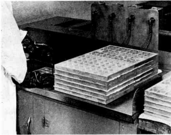
Fig. 10—Photograph of ultrasonic cleaning in production line.
