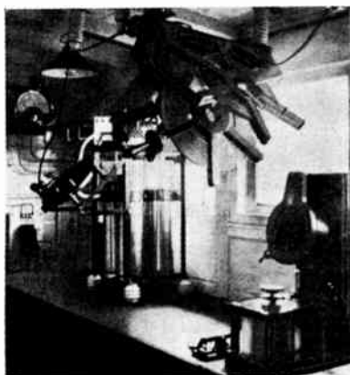
Fig. 3—Typical receiver and transmitter for shipboard in use around 1910. Receiver (right) consisted mainly of the coupler with its hinged primary and large tuning condenser (below). Detection by crystal rectifiers, usually molybdenum.
