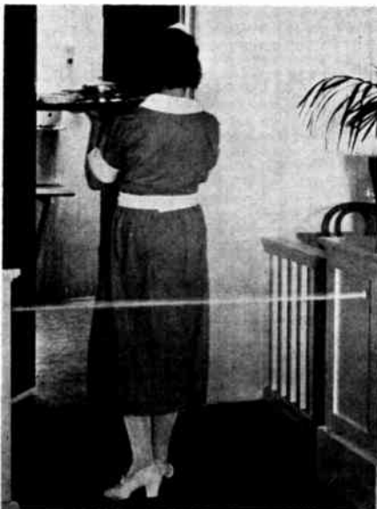
Fig. 5—Photoelectric door opener in a restaurant (1931).
