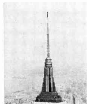
Fig. 7—The Empire State Building tower with seven television transmitting antennas.
