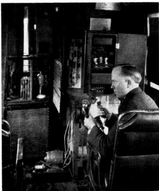
Fig. 1—Early carrier current equipment installed in a trolley car (1927).
