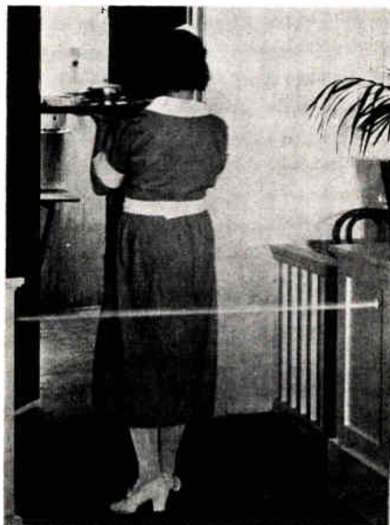
Fig. 5—Photoelectric door opener in a restaurant (1931).
