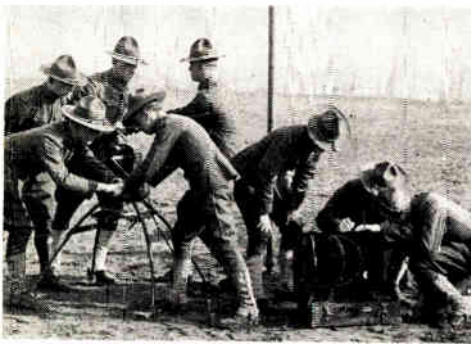
Fig. 7—Signal Corps field set developed during World War I. A spark set powered by hand-driven generator.
