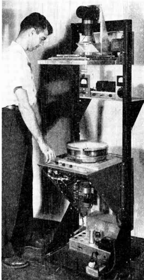
Fig. 7—Optical test stand to check Deflectron circularity.
