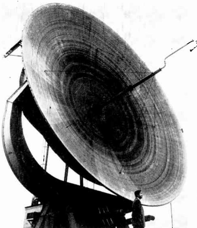
Fig. 6—Antenna used in obtaining radar echoes from the moon at S band.
