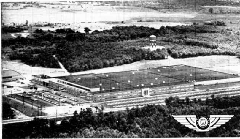
Outlined area shows addition to Air Arm's multi-million dollar facility.
