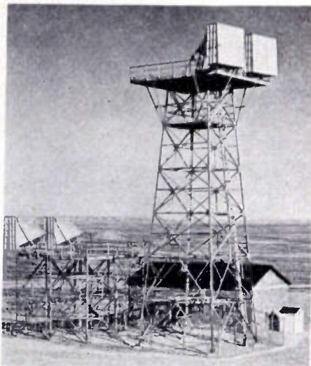
Shown above is one of a chain of 107 Bell System radio-relay stations which now link New York and San Francisco with telephone and television service. Spaced about 30 miles apart, these stations operate on a frequency of 3,700 to 4,200 mc.
