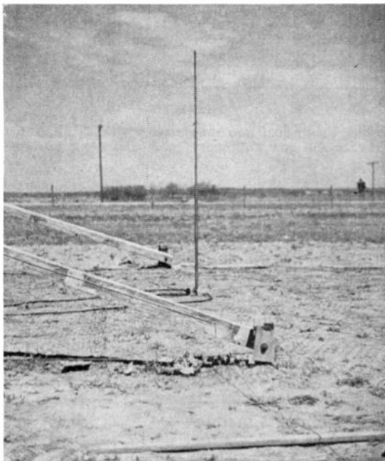
Fig. 6—The scale model of the new antenna in position between the pivot points of the "A" frame.
