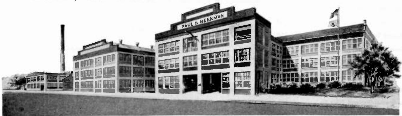
Below: Paul & Beekman plant, largest producer in the East of cans for the radio industry.
