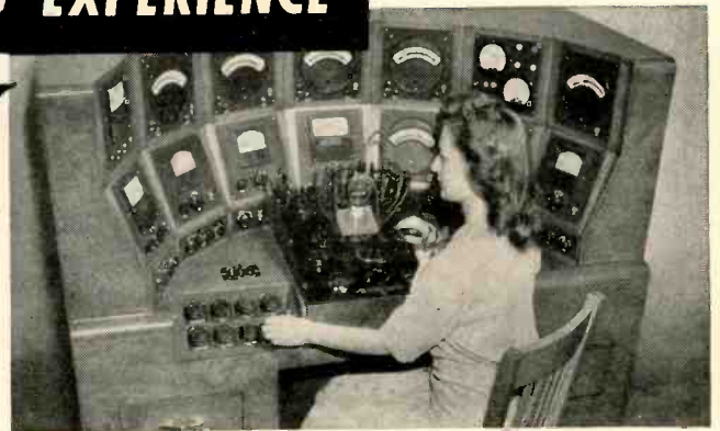
Extreme accuracy and flexibility of this Hytron master test station particularly fit it for quality control.
