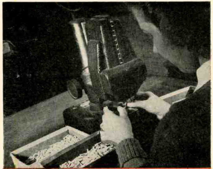
Electrolimit gauging checks dimensions to the fifth decimal.
