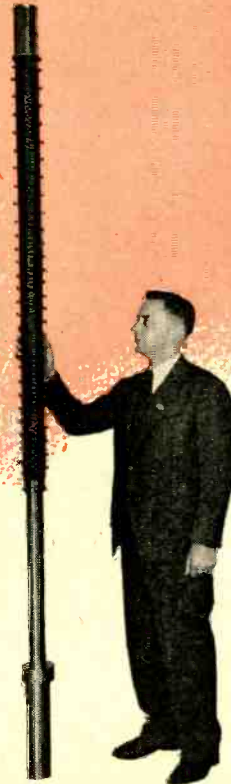
2,000,000 volt direct current precision radiographic tube, type VM
