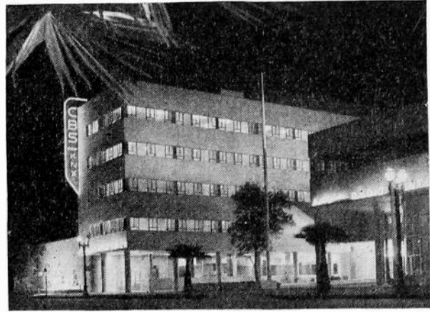
Fig. 1—Main building of CBS Studios at Columbia Square, Hollywood, California.
