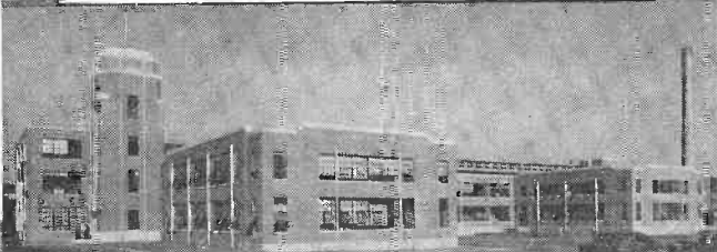
SYLVANIA RADIO TUBE FACTORY, SALEM, MASS. Another great up-to-the-minute tube plant. Daily capacity 65,000 tubes.
