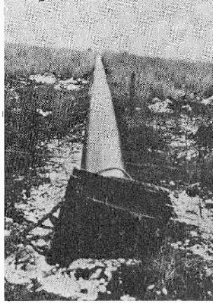
Fig. 17—The pole which was removed from the top of the original WCAU antenna. This pole was 100 feet long.
