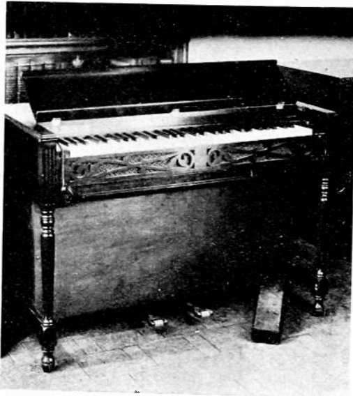
Fig. 15—Miessner electronic organ with single bank of reeds and single electrostatic pickup.
