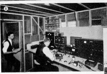
NOISE TEST—This test, made in a shielded chamber that eliminates external interference, reveals defects in internal resistor structure that cause noisy resistors. The accurately controlled Allen-Bradley processes result in such uniformity that quiet resistors can be consistently quaranteed.
