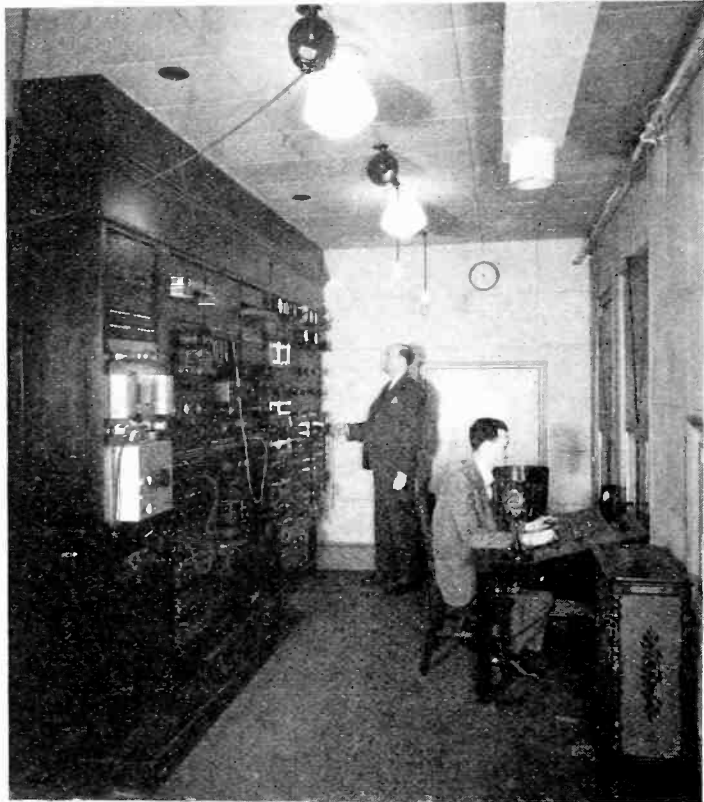
Fig. 12—Control room, Times Square Studio, New York.
