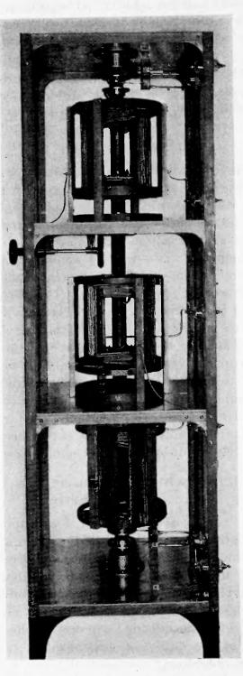
Fig. 13-Side view of the goniometer used with the polydirectional radio range.
