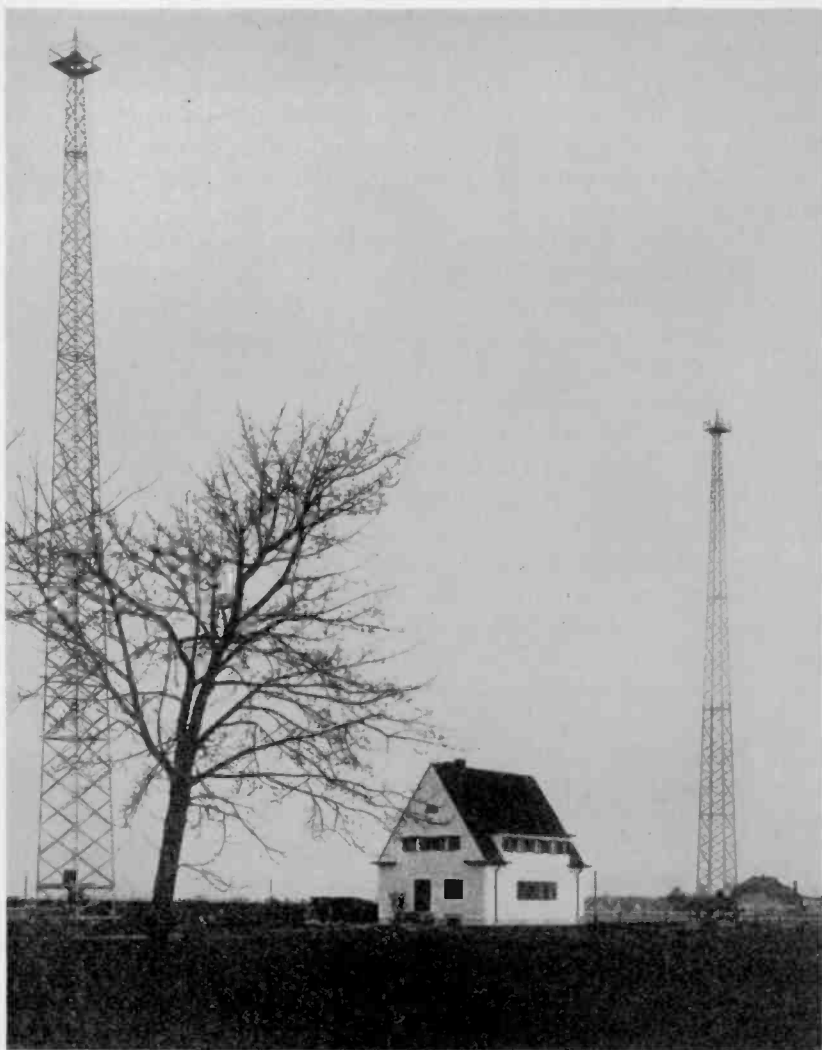
Fig. 11—Nurnberg airport transmitting station.
