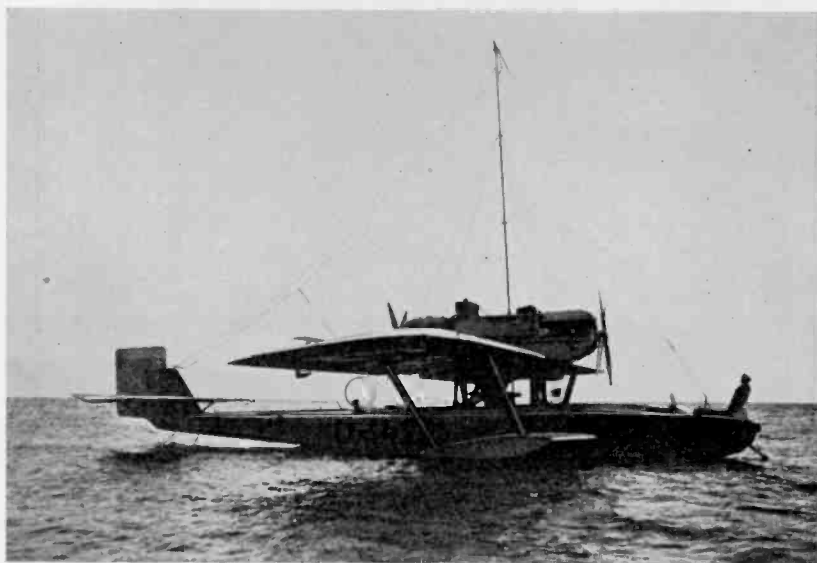
Fig. 25—Dornier Wal with emergency antenna and compass loop.
