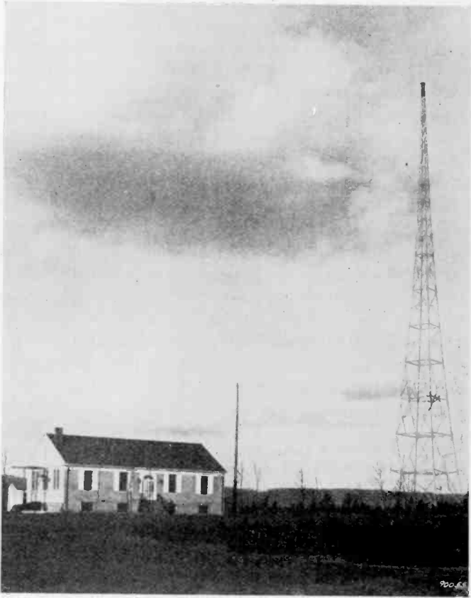
Fig. 9—General view of transmitter house and one of the antenna towers, Station WJZ.
