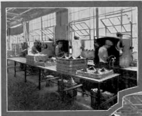
Above: A section of the Cone-spraying Department where the cones are water-proofed prior to assembly.
