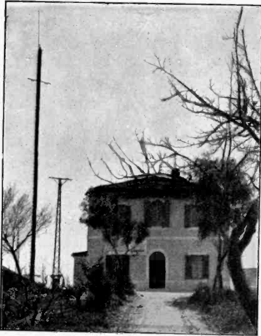
Fig. 4—Outside View of the Monterotondo Receiving Station.
