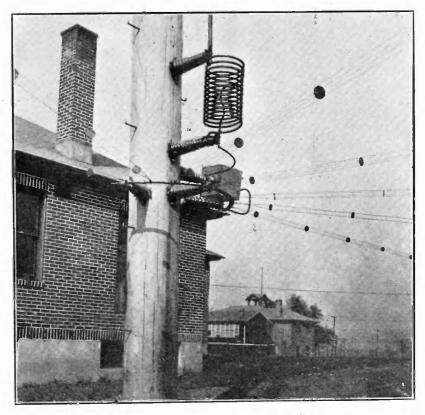
FIGURE 3-Antenna Loading Coil and Ammeter
