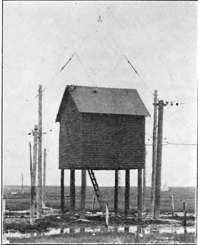
Tuning House at End of Transmission Line, Located 1,400 Feet from the Transmitter in Power House, Tuckerton, N. J.
