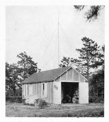
FIGURE 5—Receiving Test Station Near Riverhead, L. I., Showing Vertical Antenna Projecting Through Roof of Building
