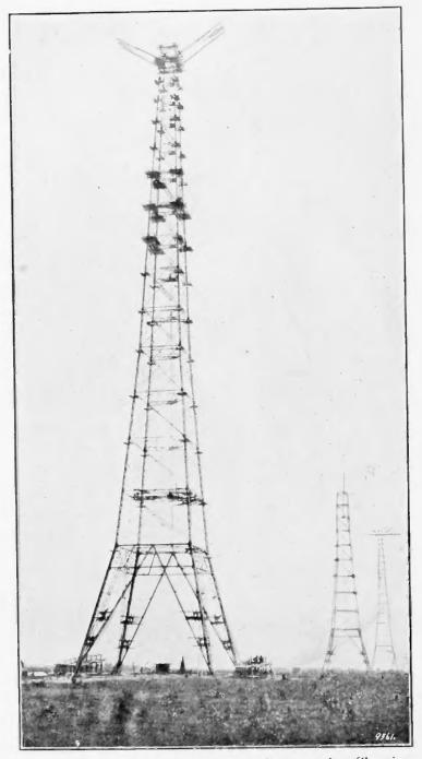
FIGURE 2—Three of the Towers in Construction Showing Cranes for Hoisting 75-foot Cross-arm Sections 573
