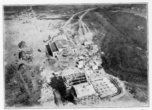
FIGURE 4—Aerial View of Radio Building and Power House Taken From Top of Tower Nearest Station; Taken During Construction of Buildings
