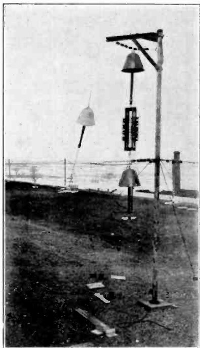
FIGURE 13—Counterpoise and Outdoor Tuning Coil at "WGY"
