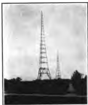
FIGURE 38—Great Lakes Station
