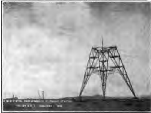
FIGURE 21—Tower Base, 350 K. W. Station, San Diego
