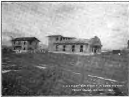
FIGURE 20—350 K. W. Station Buildings, San Diego, Cal.
