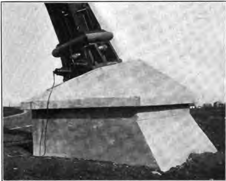
FIGURE 2—Base of Tower and Ground Switch, Arlington
