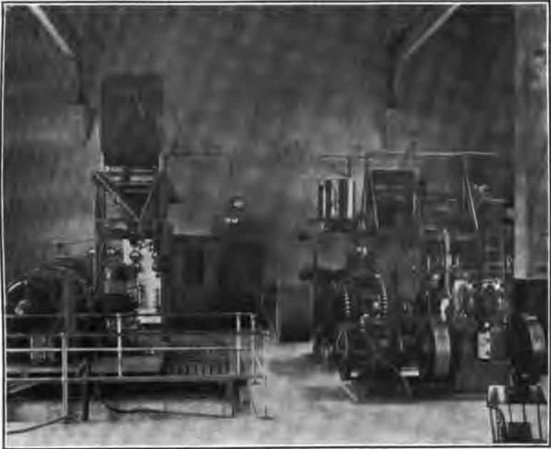
FIGURE 12—Arc and Spark Transmitters, Arlington
