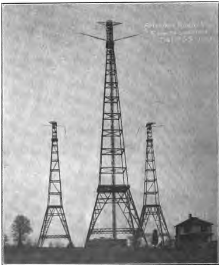
FIGURE 1—Towers and Station, Arlington
