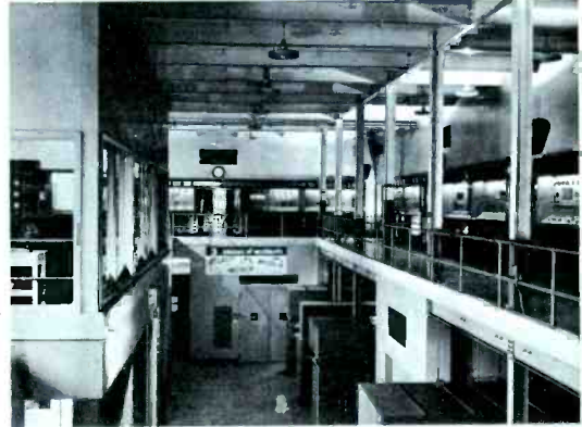
Fig. 4. Interior view of VOA's Tangier relay station showing 100-kw transmitters (upper level) and 35-kw transmitters (lower level).
