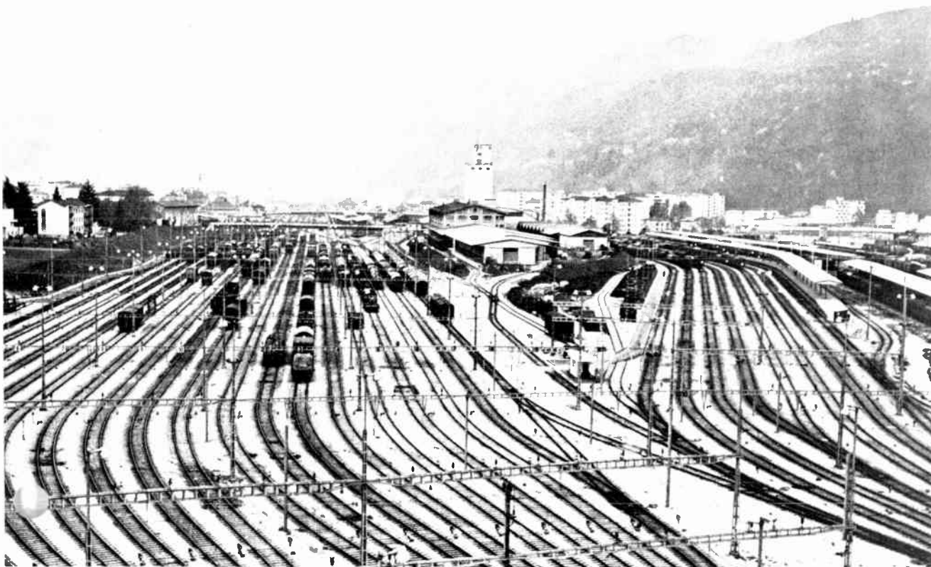
[2] View of the Chiasso marshaling yards on the Swiss-Italian border. Here, an ever-increasing degree of semiautomation in customs clearance and reassembling and routing of trains expedites the arrivals and departures of international trains.
