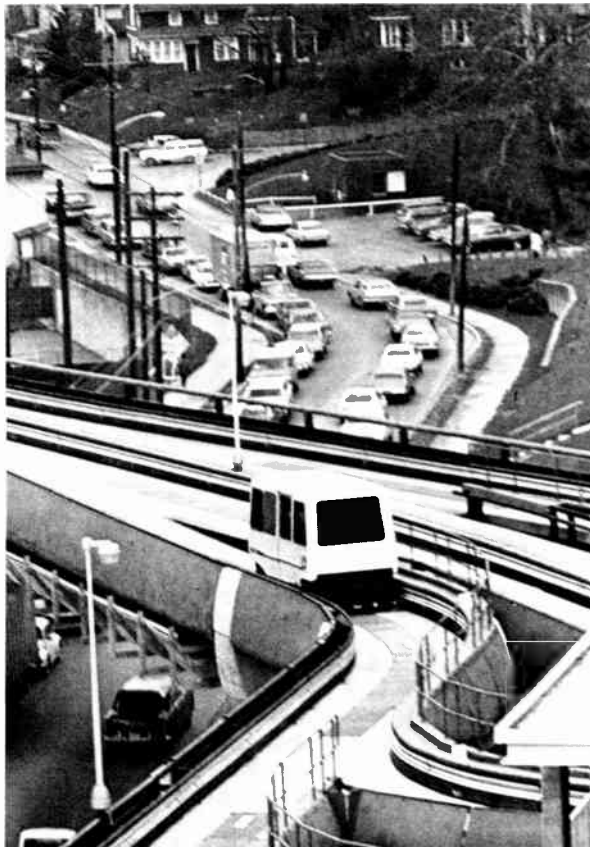
[4] Bird's-eye view of the Morgantown experimental PRT guideway and typical vehicle, along an elevated portion of the 11-km-long line financed by DOT's Urban Mass Transit Administration.
