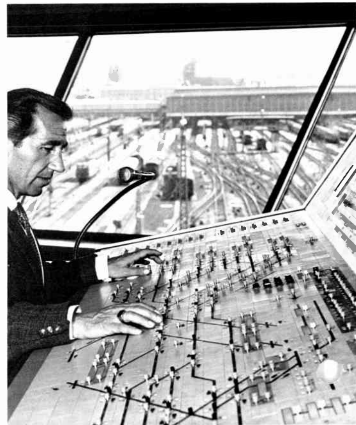
[3] From Munich's Main Station signal cabin, about 1000 train, 5000 shunting, and 600 locomotive operations are controlled daily by a sophisticated CTC system. Formerly, this same quantity of operations had to be handled by 11 cabins, five block posts, and one junction location.
