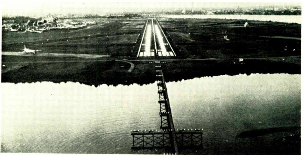
FIGURE 2. Pilot's view of a landing approach on an illuminated instrument-landing system (ILS) runway at the Washington (D.C.) National Airport.
