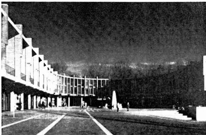
FIGURE 7. View of the horseshoe-shaped shopping plaza in Lake Anne Village, Reston, Va. One in a series of “new city” concepts, Reston is an excellent example of the merger of art and technology in design and construction.
