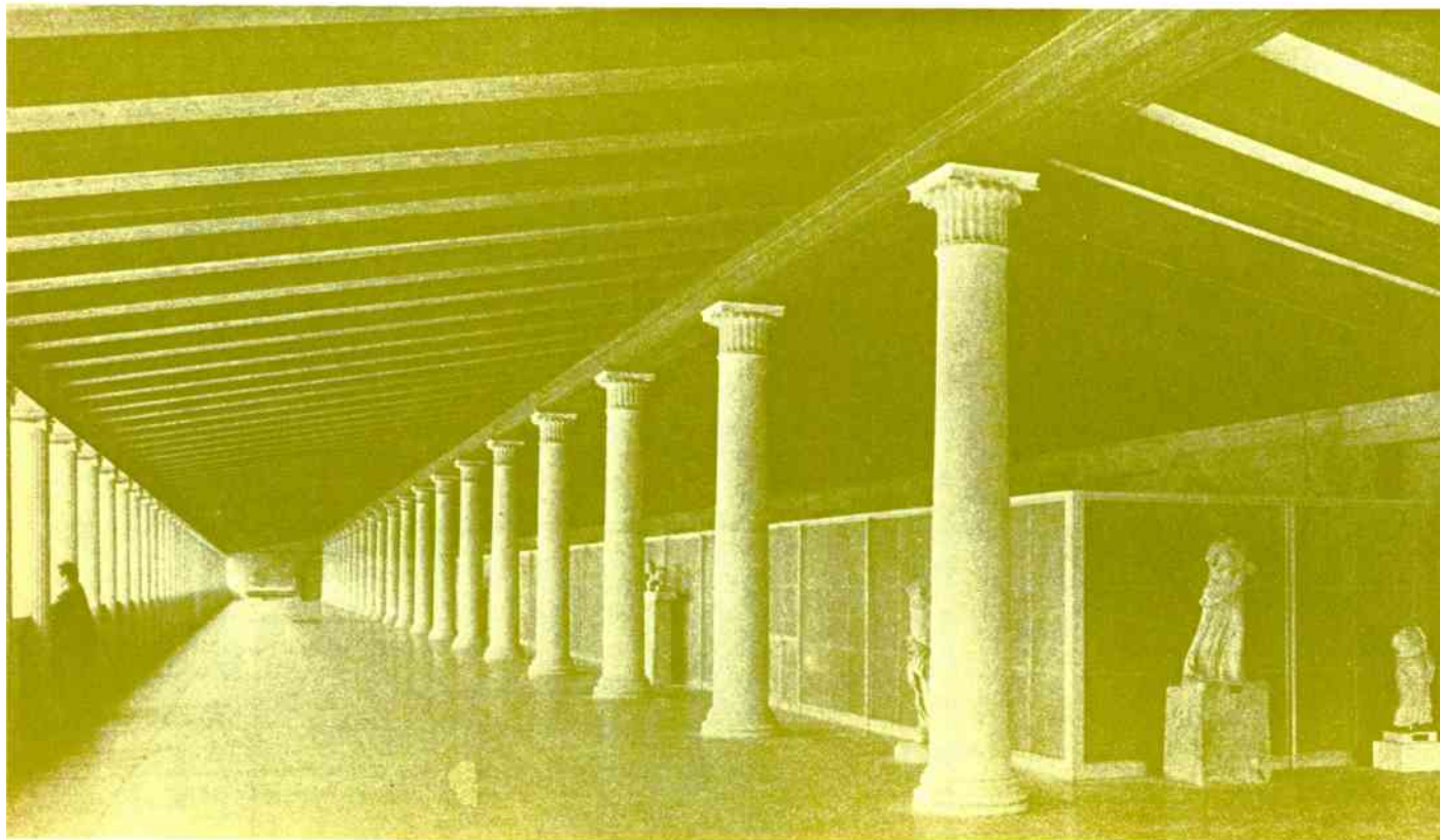
FIGURE 1. The ancient stoa of Athens, as reconstructed by precise modern archaeological techniques, is an excellent example of the beautiful proportionality of Greek post-and-lintel design and construction.
