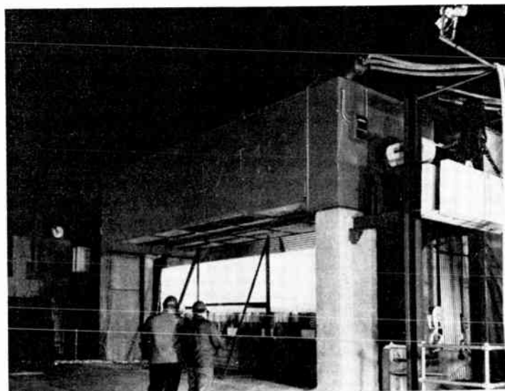
FIGURE 8. 60-Hz induction-heating installation. The slab is lifted into the heater coil.
