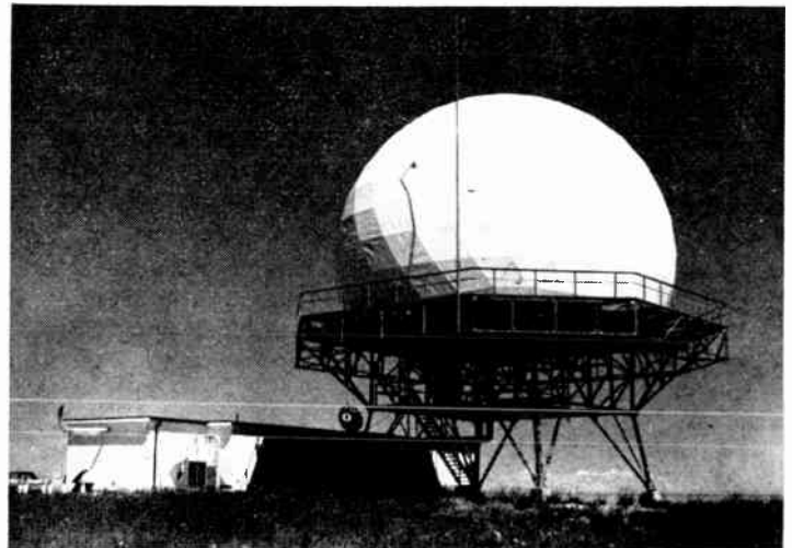
FIGURE 5. FAA Air Route Surveillance Radar facility at Parker, Colo., near Denver. (Courtesy Denver Area Office, Federal Aviation Administration)
